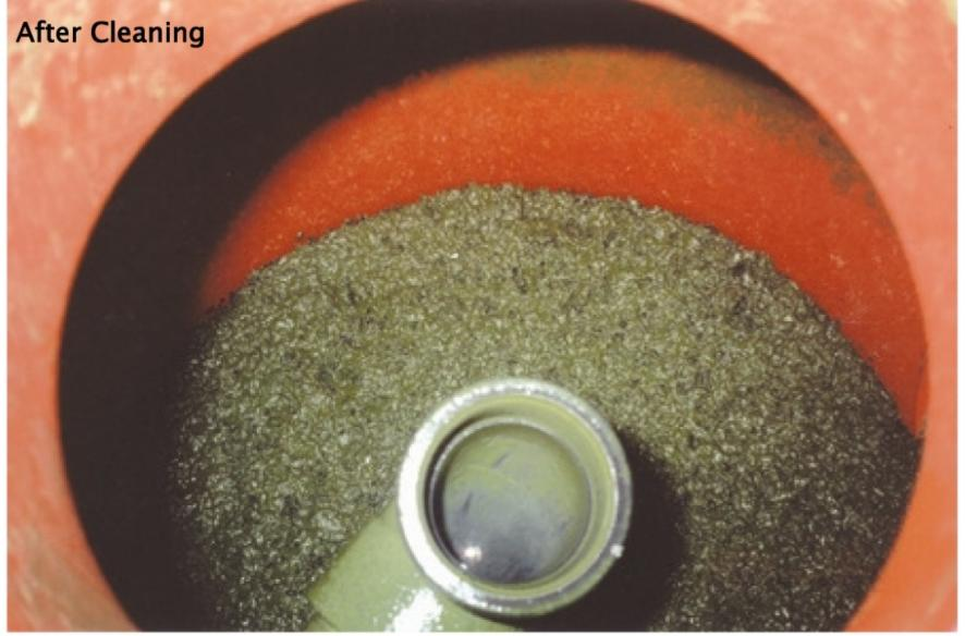
To clean, TRIPLE 7 Colloidal Concentrate was added to the media filter, then the back-wash cycle was run constantly recycling for approx. 15 mins, then the water was dumped. The process was repeated twice.
